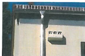
[Pic. 6]: Example of installed 1SP
